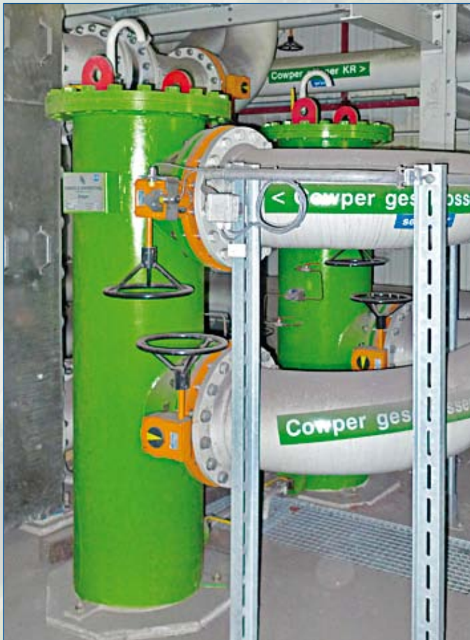
Fig. 2 Single Filter in welded steel design
