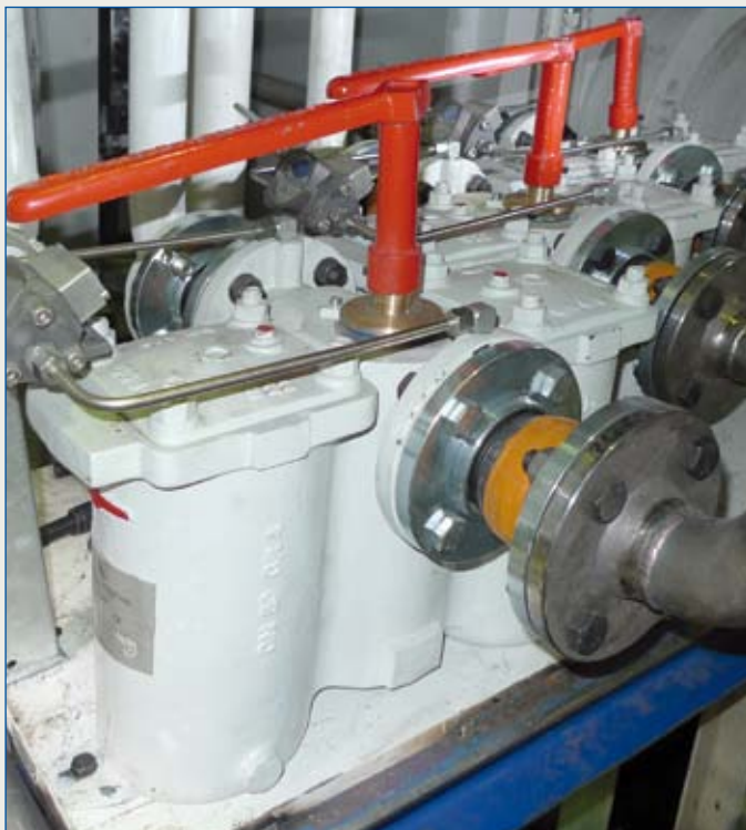
Fig. 4 Duplex Filter in cast iron design
