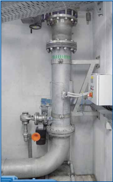
Fig. 8 sea water filtration for snow making system
