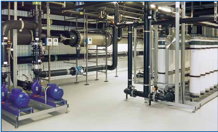
Fig. 11 drinking and process water filtration in brewery
